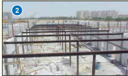
Iron skeleton before installation in wide buildings
