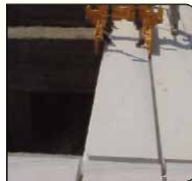
Install the slabs close to each other near the edge of the rib to form letter (U).
