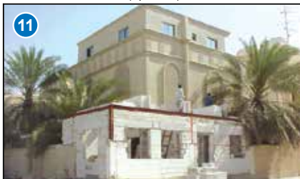
The building upon installing the slabs
