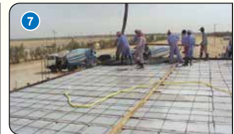
Install a reinforced steel net of 8 mm diameter (optional).
