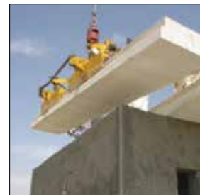
Slab Fixing
