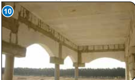
The look of slabs after installation.
