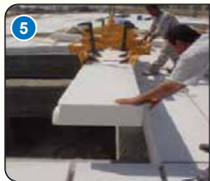
Install the slabs close to each other near the edge of the rib to form letter (U).
