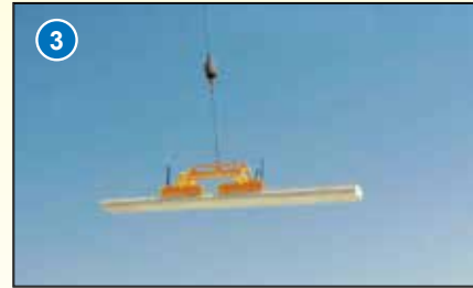
Lifting the slabs to be installed
