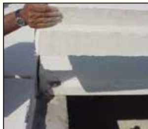
Install the slabs close to each other near the edge of the rib to form letter (U).
