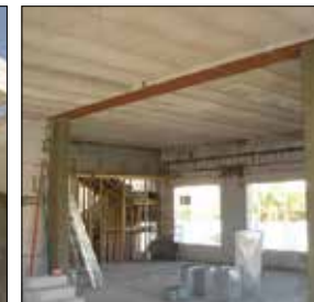
Span over 6 meter
